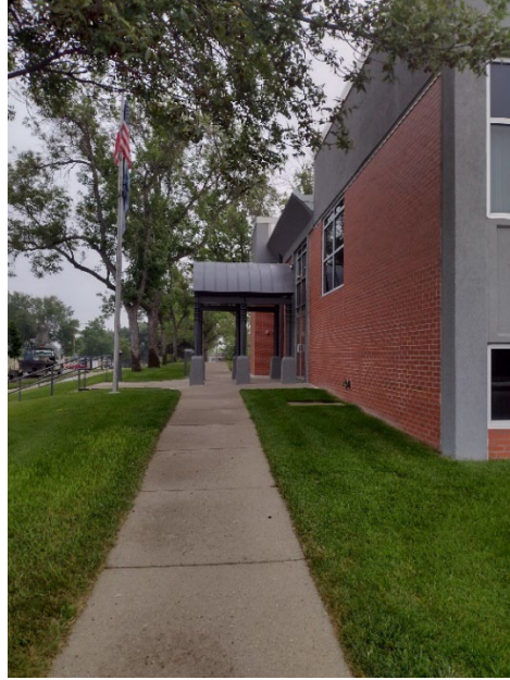
Looking North from Divide Avenue, after painting July 25, 2024
