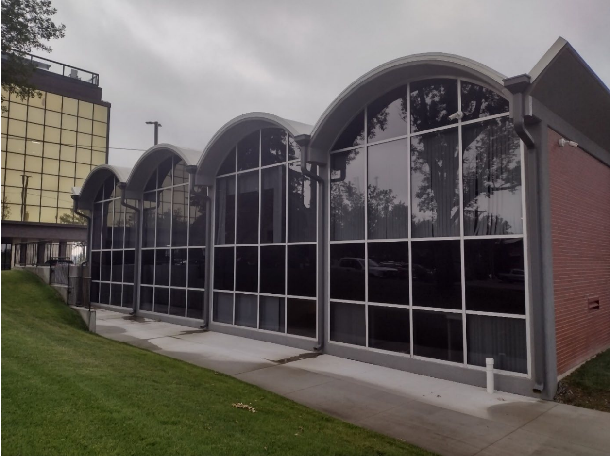
Department retaining wall on July 23, 2024. North Side of the Building Photo credit: Rick Owings
